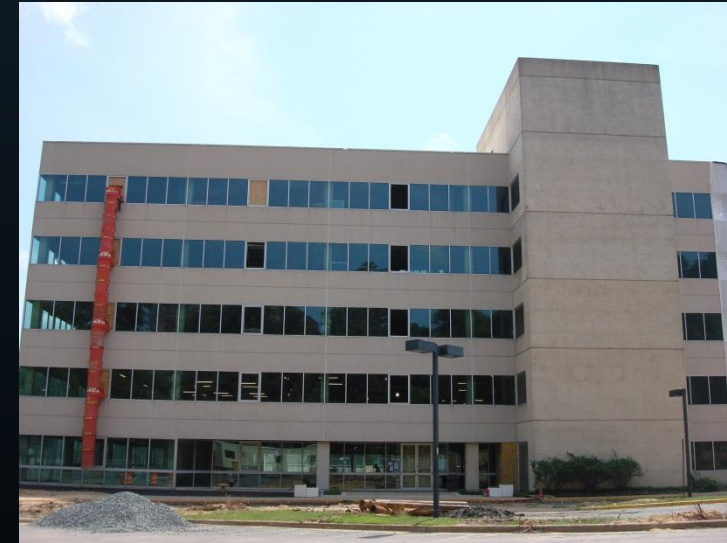
PREVIOUS WESTERN FACADE
